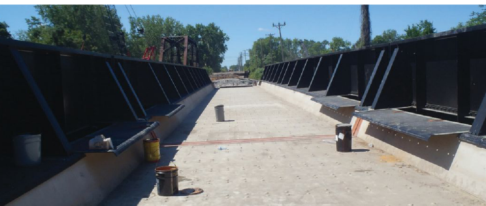
◀ A view, from the deck, of two new spans set onto new piers.
